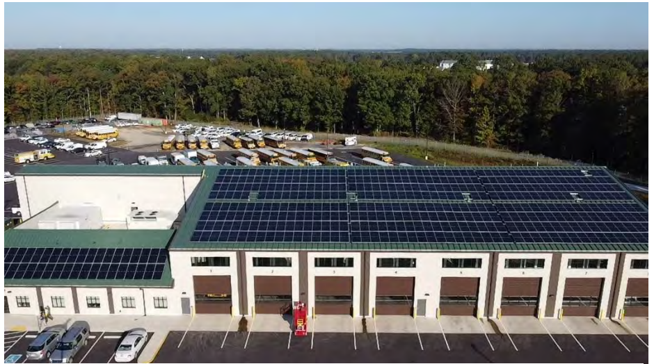
Solar on the Chesterfield Fleet Services building. Source: Chesterfield County
